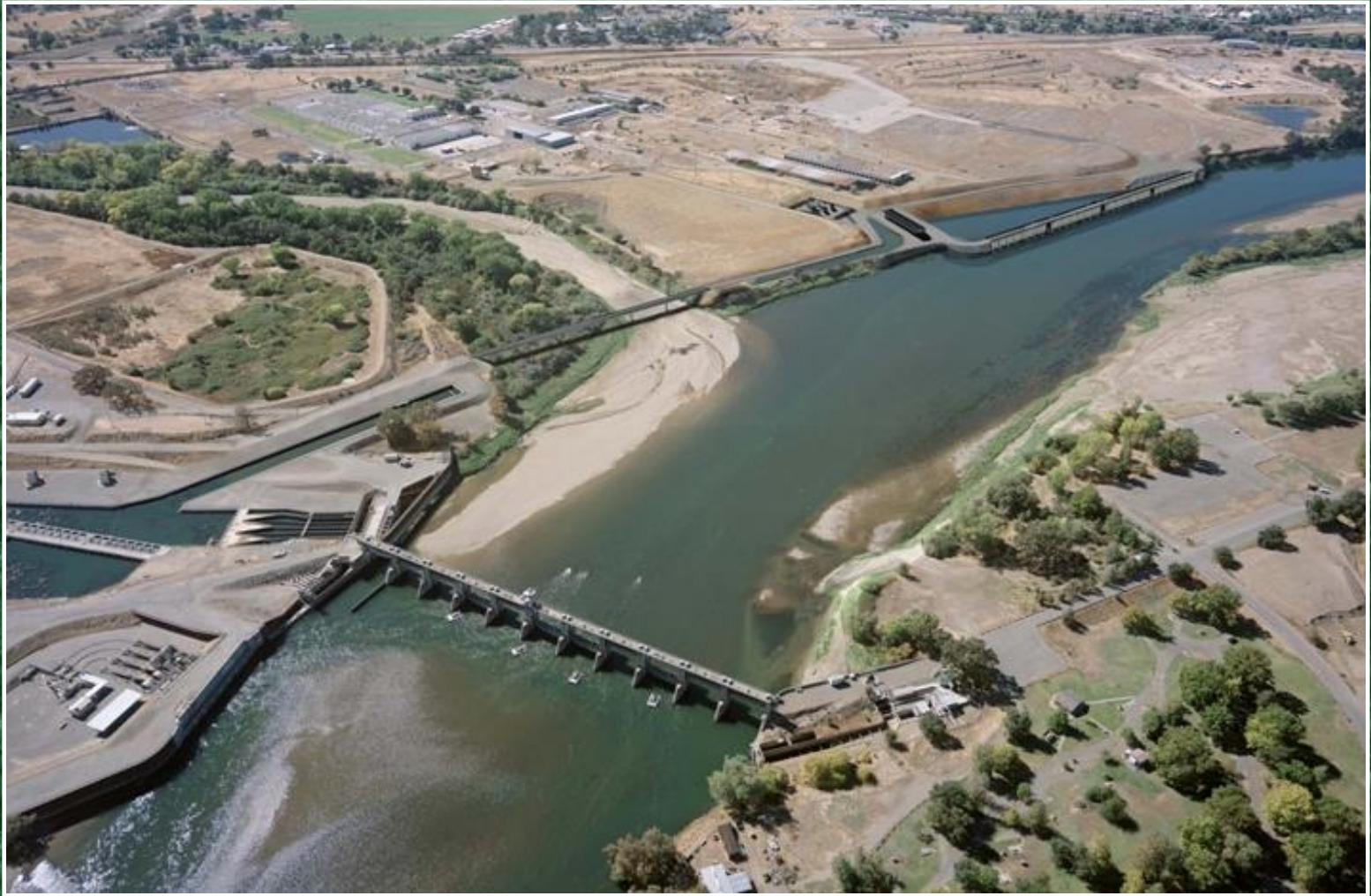
Gates Up Year Round :Permanent Pumping Plant (USBR)
