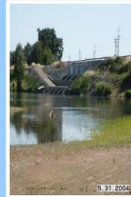
**Revegetation can be used to direct flows away from flood-control structures.**
