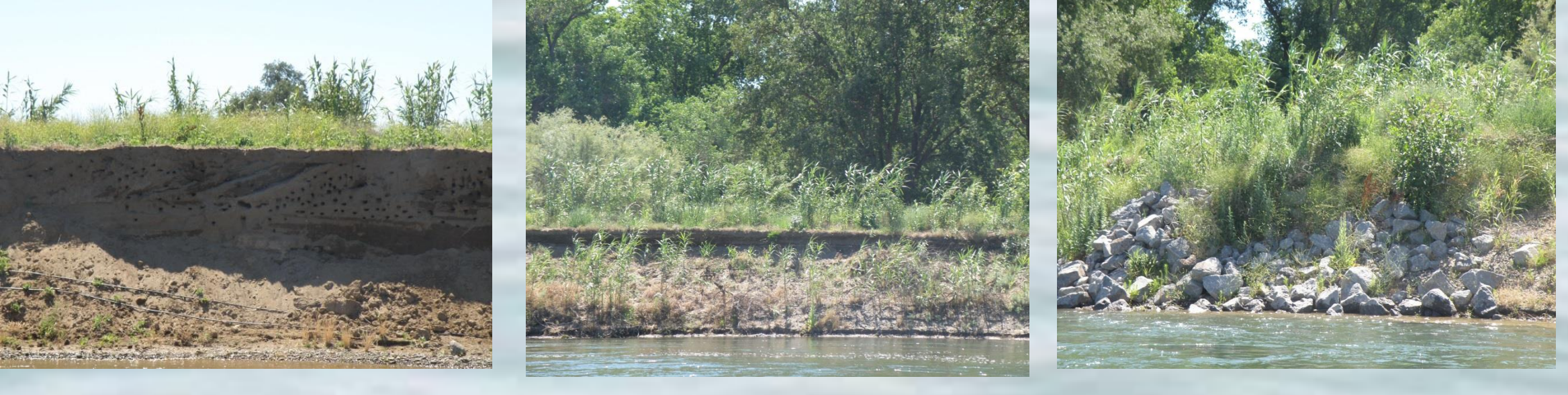
River Mile 233.5 Left— Private Bank Revetment 2012 • Irrigated Arundo donax & • Trenched rip-rap
