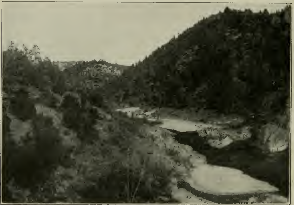
Pilot Creek Dam Site on North Fork of American River
