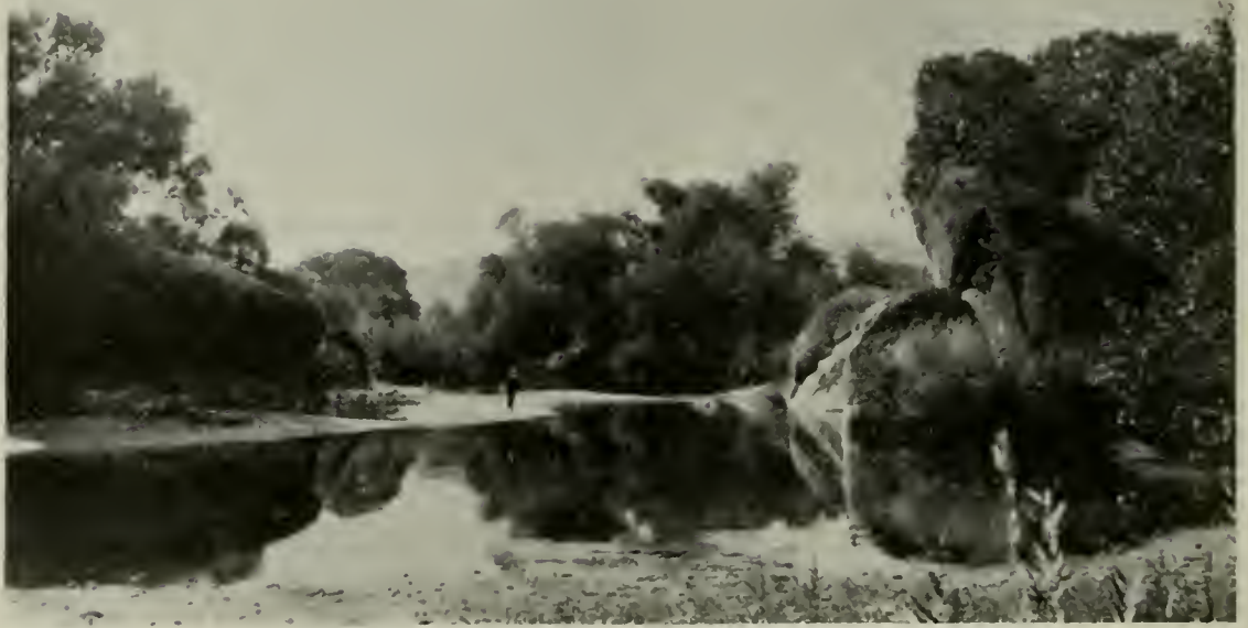
Millsite Dam Site on Stony Creek
