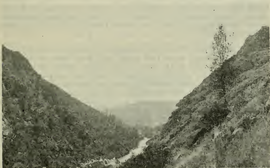
Monticello Dam Site on Putah Creek
