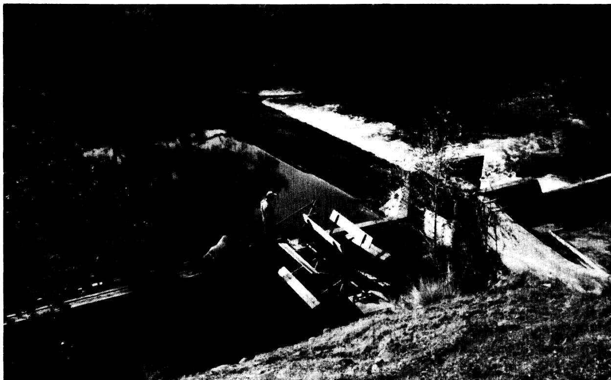
The Upper (or Company) Diversion Dam on Mill Creek has a satisfactory fish ladder and screen. At high water, fish can swim directly over the dam.
