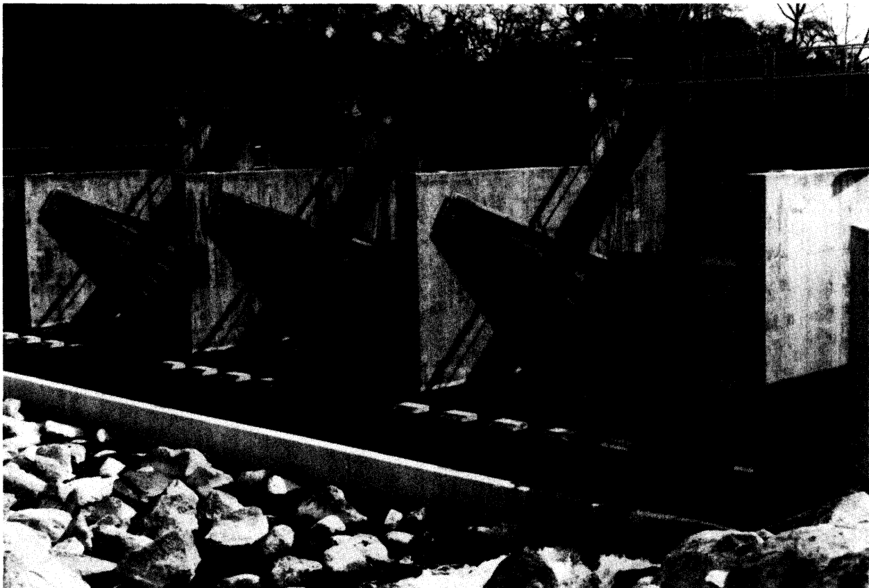
A gate structure similar to this one on Kelsey Creek in Lake County could be constructed on the Sacramento River to make adjustment of flashboards at the ACID dam easier.
