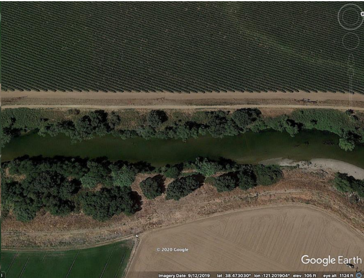
West view of banks
